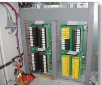
• Manual control panel for Archer Batching System
