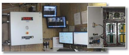
• Concrete control panel for Archer Batching System
